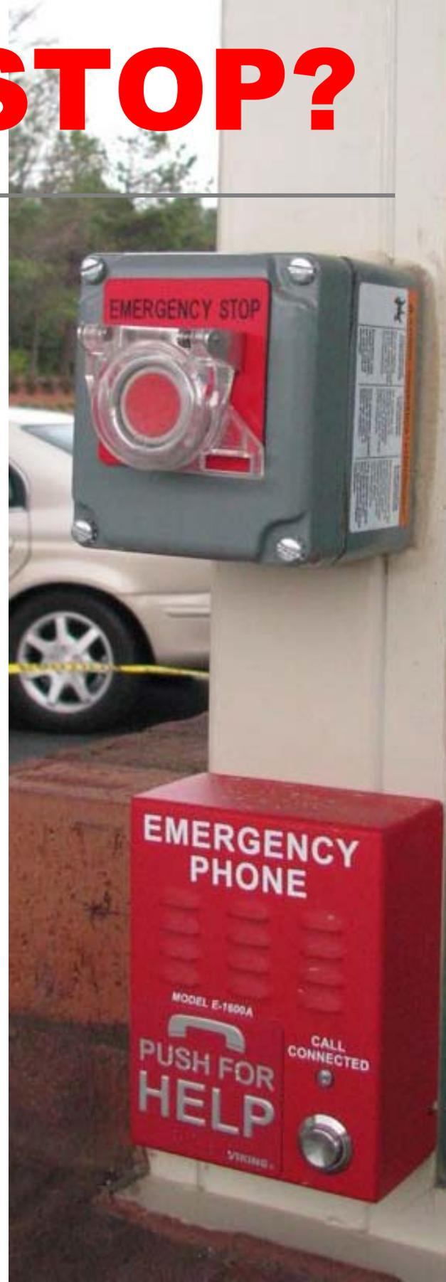
The “EMERGENCY STOP” (E-stop) system at a gas station is a safety system installed to safeguard persons and property against the potential of a shock or fire.
