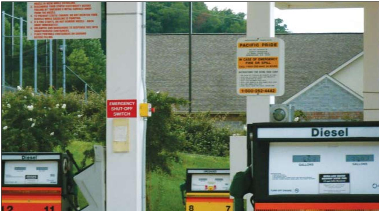
Photo 1. Emergency shut-off switch located within 30m (100ft.) of a fuel dispensing device which it serves.
